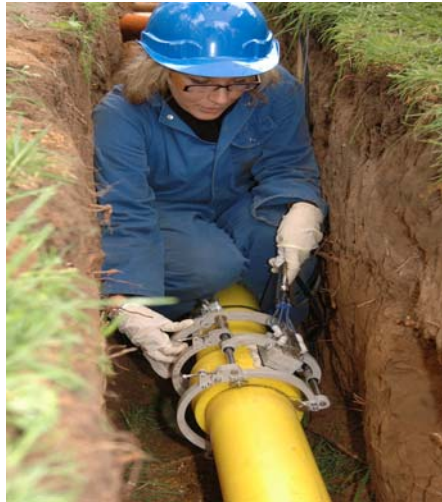
Figure 11 Prototype of ultrasonic inspection manipulator operated in field conditions at TWI.
