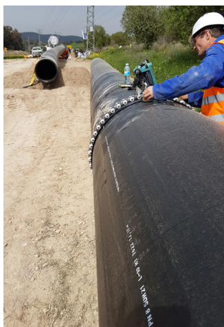
On-site PE pipe joint inspection
